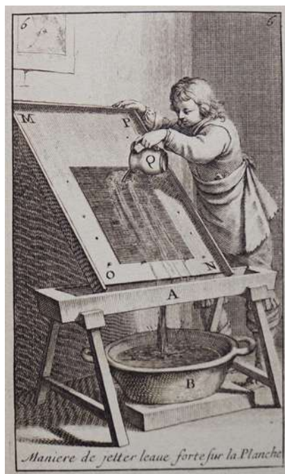
Method of pouring acid onto the plate (A. Bosse, 1645)
